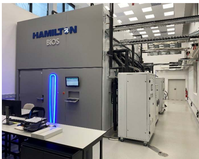
Figure 1: Bios – biobanking facility
